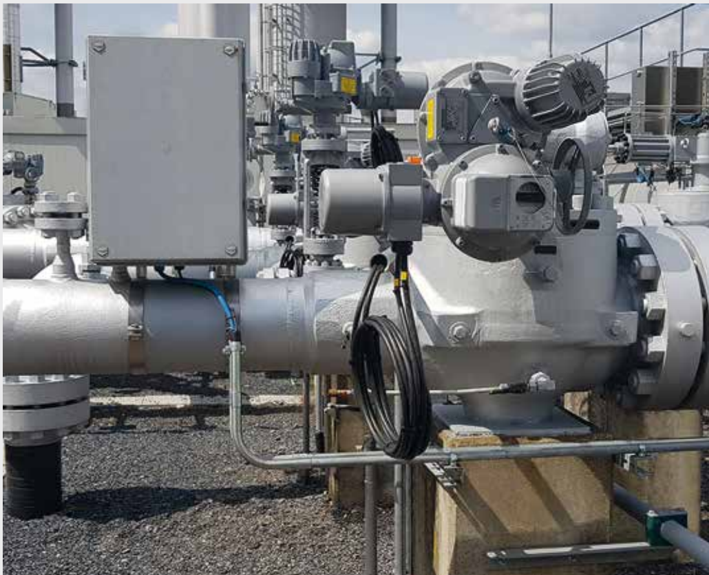
Top entry ball valve installed at Uniper gas storage site
